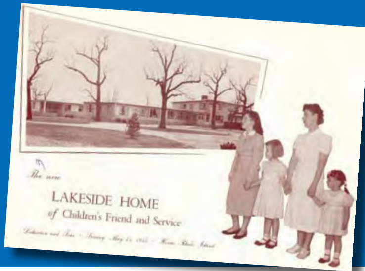
The new Lakeside Home.
